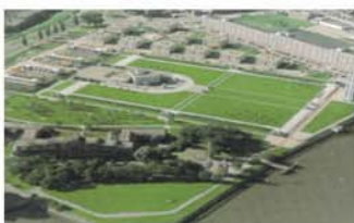
Reusing inner city docks to bring a waste water treatment plant underground (Dokhaven, Rotterdam, the Netherlands).
