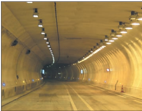
Figure 4 - Section courante du tunnel
